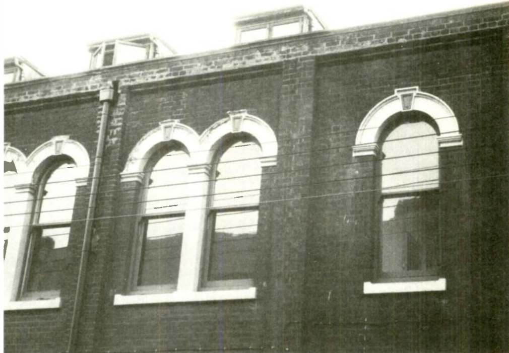
Low voltage, high current cable runs can induce large fields at bedroom height.
