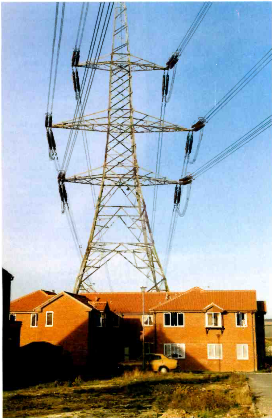
The UK: new houses are built under power lines
